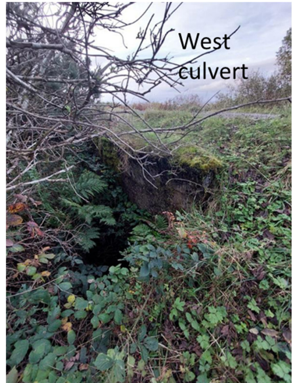
Photo of existing WCC6a, western culvert 27/10/2022.
