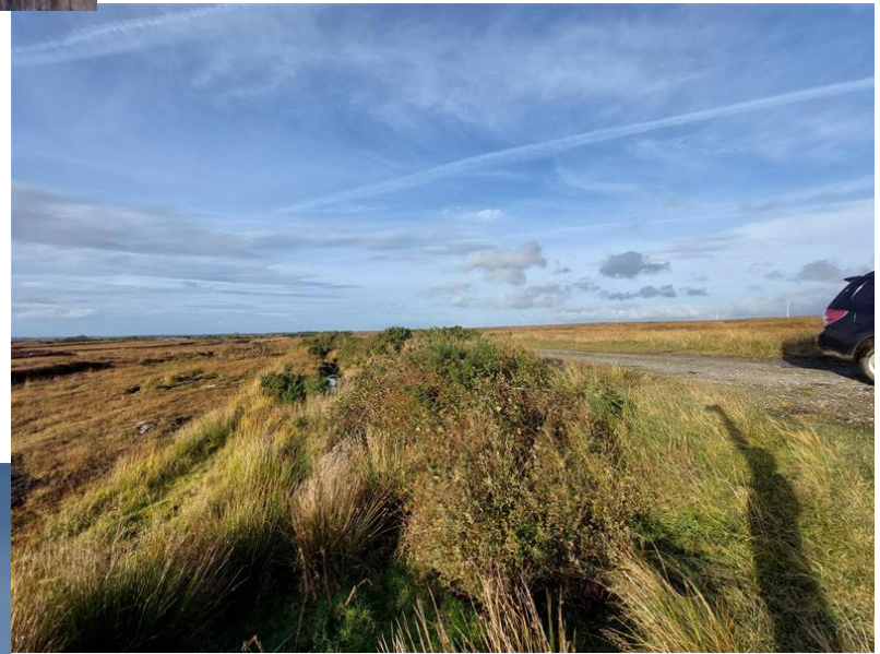
Location of WCC7, no existing culvert, drain runs to north either side of track 27/10/2022.
