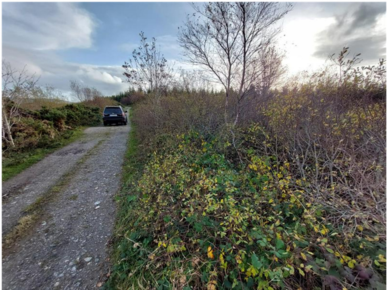
Photo taken looking south , bump in road at car is culvert. Drains converge (north flows south, south flows north to culvert and off to the west 27/10/2022.
